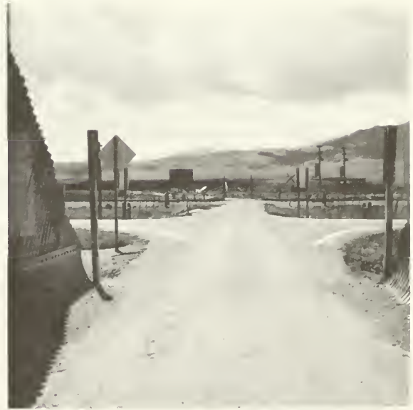
Looking West from WEST ENTRANCE
